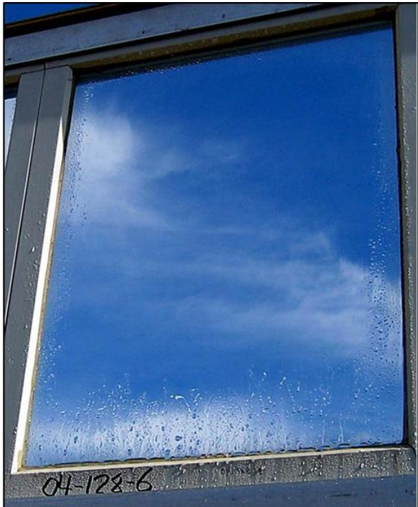
Fig 03: Silicone glazing residue causing picture framing (beading of the water due to silicone residue)
