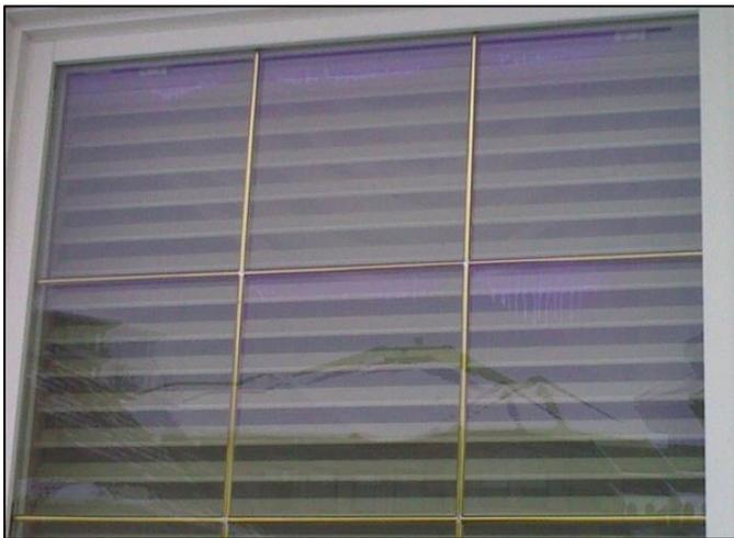
Chemical fogging as seen in a non-Cardinal IG produced unit. Chemical can be seen running down glass in area of internal grills
