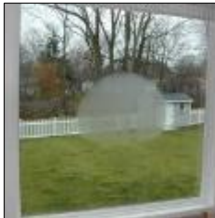
Fig 01-3: Condensation Ring
