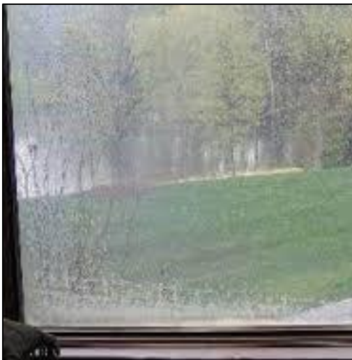
Fig 01-1: Airspace Condensation
