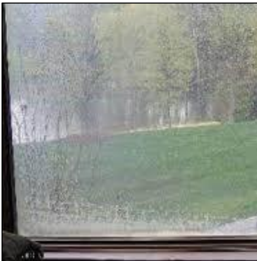
Fig 01-1: Airspace Condensation
