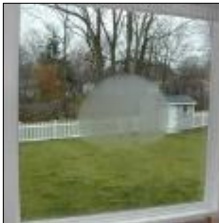
Fig 01-3: Condensation Ring
